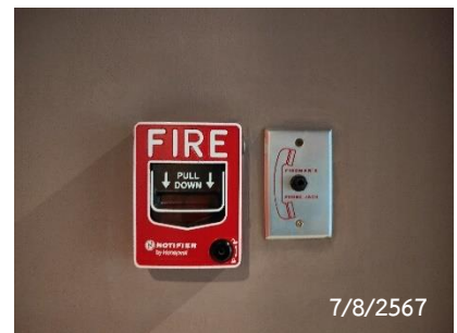
Fire Alarm Manual Station
