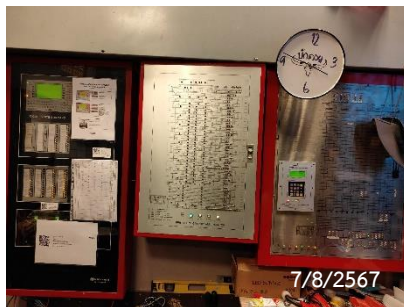
Graphic Annunciator Fire Alarm System
